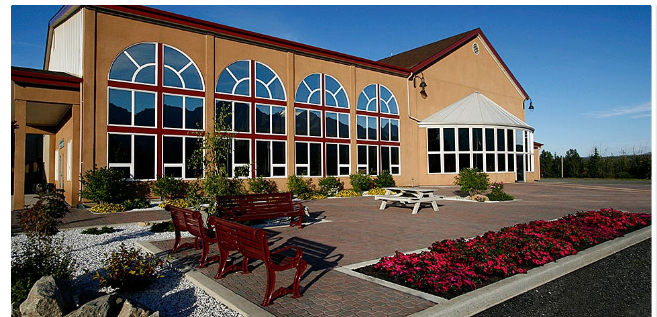
St. Elias Convention Centre Photo Credit: Yukon Convention Bureau
