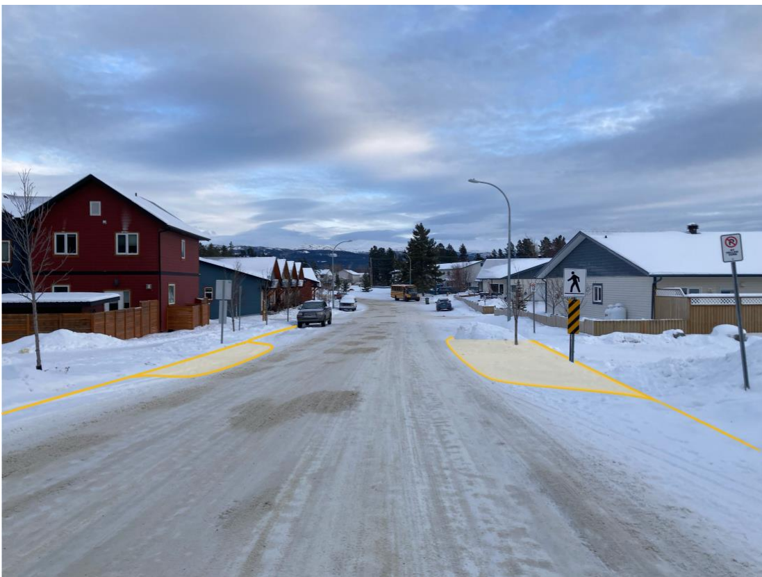
FIGURE 11: EXAMPLE OF CURB EXTENSION IN TAKHINI NORTH NEIGHBOURHOOD AND WINTER SNOW MAINTENANCE (BUILT-IN 2009)
