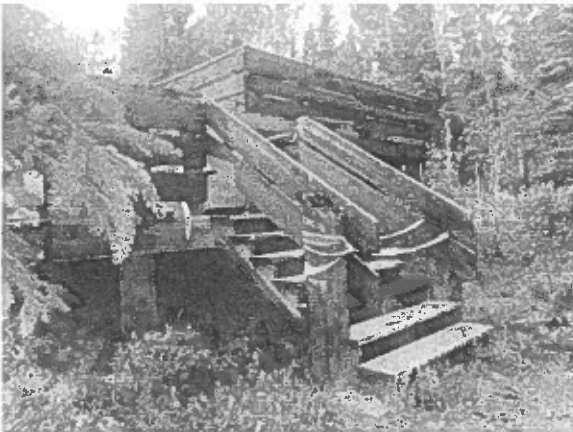
East entrance to viewing platform.
