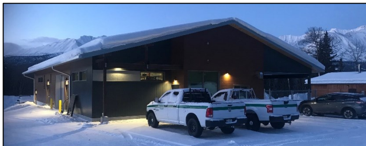
The Kluane NPR Trades Building has Dark Sky friendly full cut-off light fixtures, for light only where needed.
