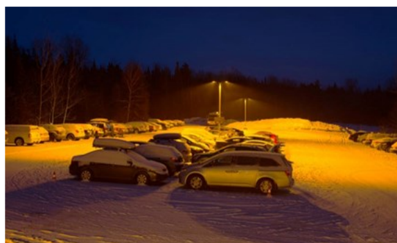
Compliant – Mont-Megantic AstroLab parking, features full cut-off amber LED lighting.
